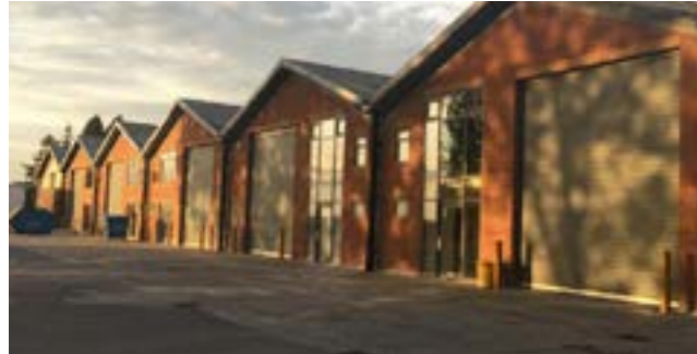
High Bay Units - Aldridge, West Mids.
