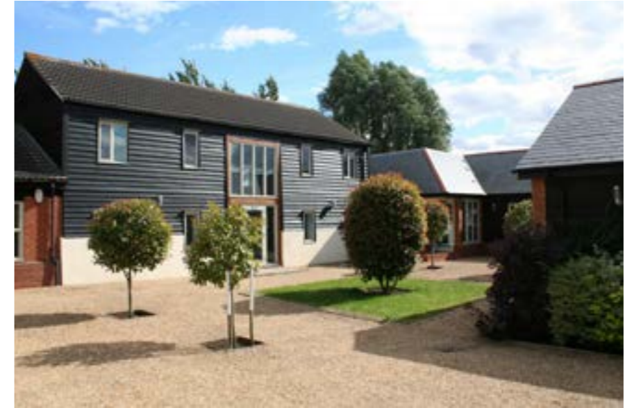
Downstairs office / Studio space
